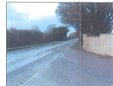
PHOTO 1 - VIEW TO RIGHT FROM EXISTING ACCESS
